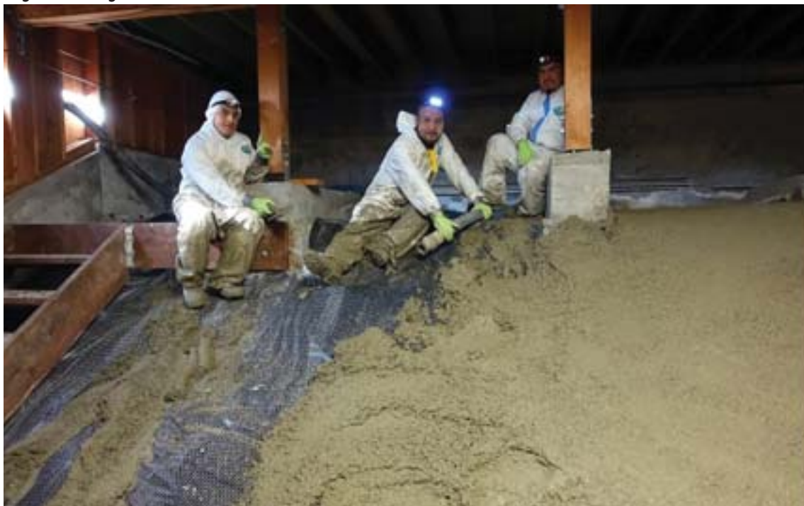
Pouring concrete over crawl space, especially on an underground incline, is hot and dirty work.
